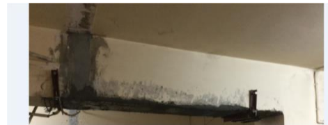
Beam strengthening
