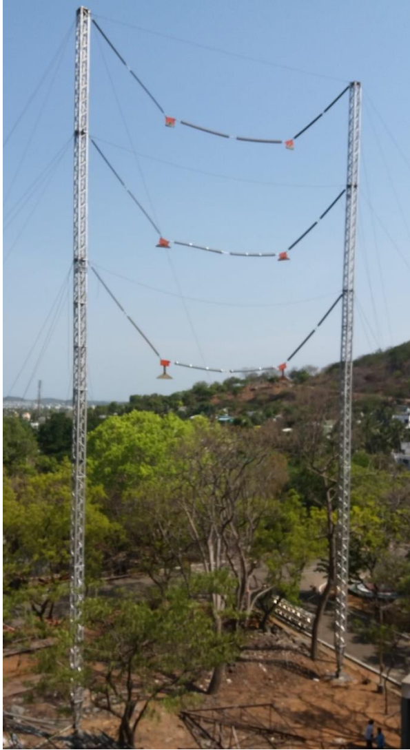
Typical view of the ERS developed
