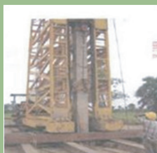
Fly ash Concrete Mixes for Thermal Power Project
